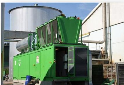
The CHP rates at 1'131 kW<sub>el</sub>. And has an excellent efficiency with  $\eta_{el}$  42,1 % and  $\eta_{therm}$  42,3 %. The CHP module is installed in a noise-protected 40” container.
