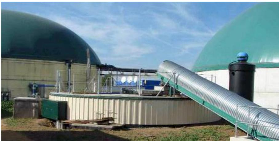
There is a straw/silage storage with 6'000 m<sup>3</sup> volume. Manure is delivered directly into the hydrolysis unit (200 m<sup>3</sup>) where it is mixed with the straw/silage that is being chopped and fed automatically into the unit. The unit is heated up and there's an aeration system to support the formation of enzyme building bacteria to turn the cellulose into glucose.
