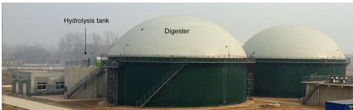
Typical FBI Chinese biogas plant running with pure corn and wheat straw. The Chinese plants have 1 to 6 hydrolysis tanks (350 m<sup>3</sup> each) and up to 8 digesters (up to 8'700 m<sup>3</sup> each).
